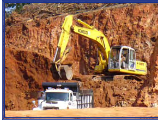
Excavator powered by used veggie oil.
