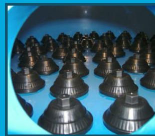
APW Double Chamber Media Filter
